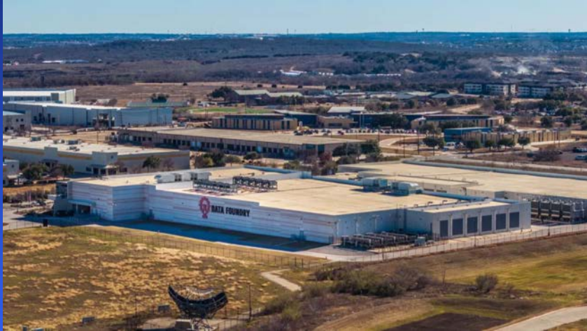
Musk Data Center in Memphis
