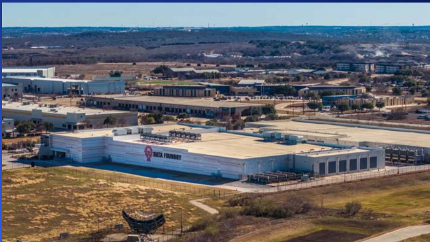
Musk Data Center in Memphis
